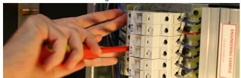
The control module installation is now complete. The lighting/load groups can be terminated into the module's output terminals.
