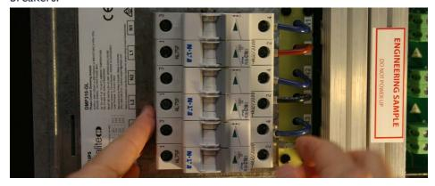
6. Terminate the corresponding Module group of the wiring loom into the left side of the circuit breakers.
