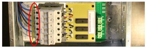
7. Recheck all terminal screws and tighten.
