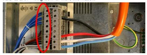
6. Recheck all terminal screws and tighten as needed.
